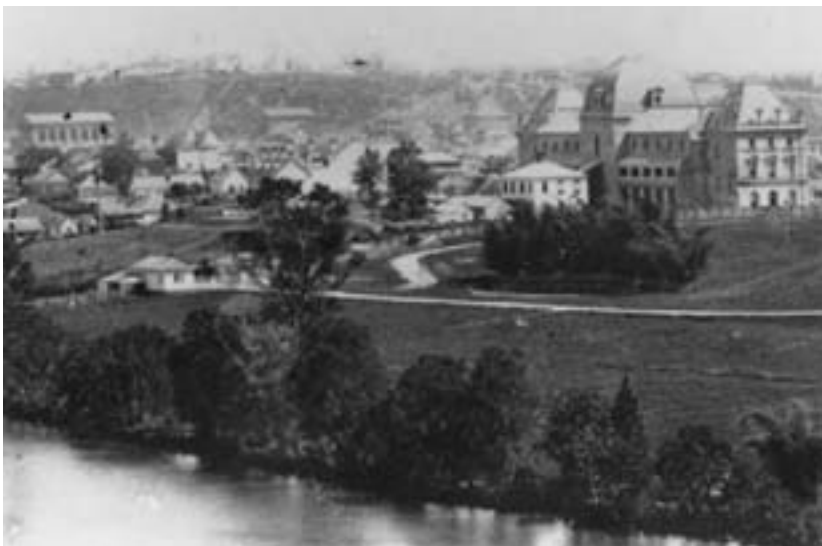
Figure 20: Rear view of Parliament House, ca.1870, showing the rear verandahs and the detached, timber refreshment room. The refreshment room faced the western sun, causing Members to complain that when they went there to get cooked meals, they themselves were cooked.
