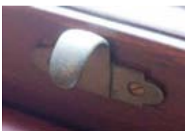
Figure 181: Original sash lift in the George Street wing
