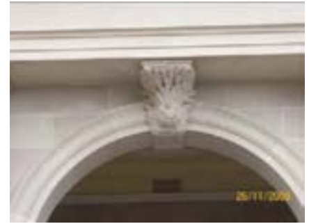
Figure 63: Staghorn keystone over the main entrance of the Alice Street wing
