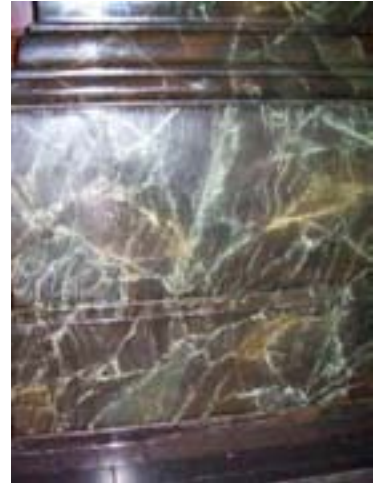
Figure 193: High quality marbling in the main entrance hall carried out by craftsman Keith Pollard in the 1980s renovations
