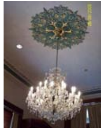
Figure 141: Ceiling rose in the original Speaker's Office of particularly ornate filigree plasterwork. The chandelier probably dates from the 1950s.
