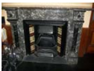
Figure 159: Black marble chimneypiece in the Dining Room with tiled register grate
