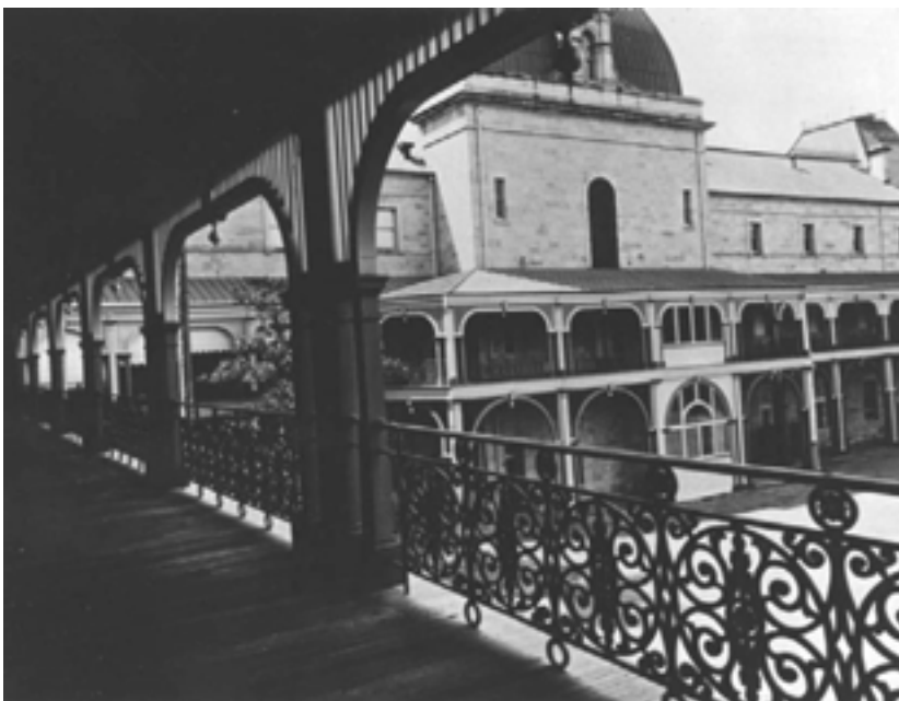
Figure 78: The back verandahs in 1950, showing the original cast iron balustrade and timber enclosure behind the grand staircase
