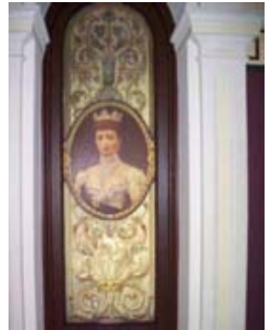
Figure 186: Princess of Wales window. The stained glass is in large panes, the only lead comes being around the portrait. Some of this may be original glass by Chance Bros.
