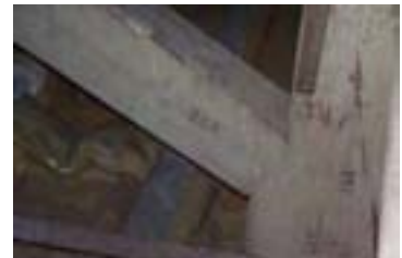
Figure 112: Carpenters' marks on the roof framing
