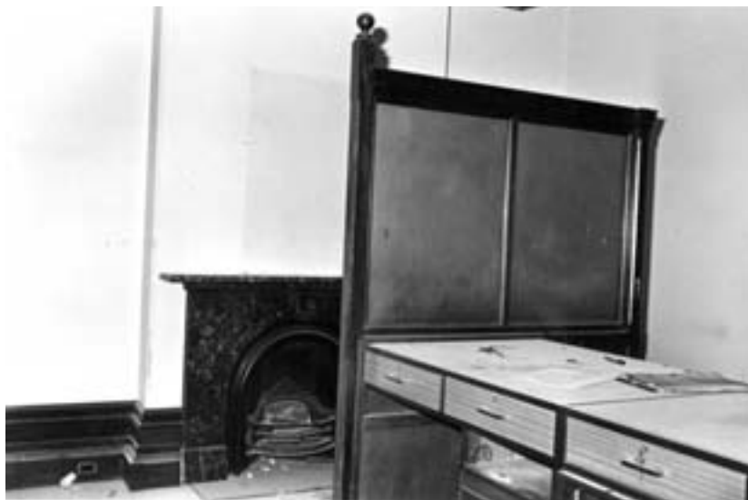
Figure 264: Small committee room in the George Street wing which was used as a post office, photographed in 1979. This chimneypiece has now been replaced with another of white marble from elsewhere in the building.
