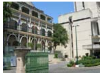
Figure 103: View of the south western end of the Alice Street wing showing its relationship to the Annexe on the right
