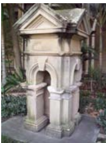
Figure 105: Some of the pinnacles removed in 1969 have been salvaged and stand in the Speaker's Green
