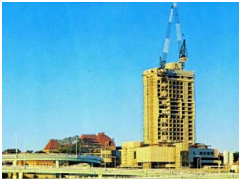
Figure 87: Parliamentary Annexe under construction
