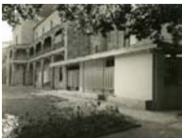
Figure 82: The rear of the building in 1957, showing a toilet block added behind the east tower
