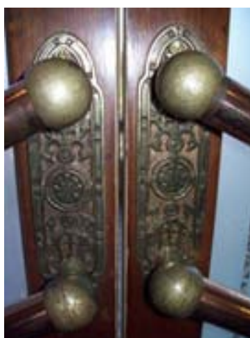
Figure 183: Handles to the Legislative Chamber and anteroom doors with matching relief pattern. The date of these is uncertain. They appear to be early but have been used on doors which were not installed until the 1880s.
