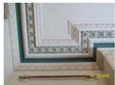
Figure 142: Cornice in the original Speaker's Office with the flowered border and a picture rod below on early patera
