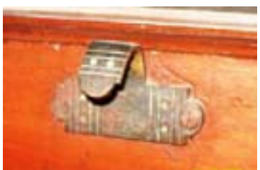
Figure 182: Original sash lift in the Alice Street wing
