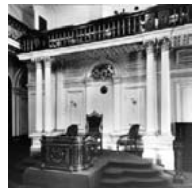
Figure 16: Reporters' Gallery above the Speaker's Chair in the Legislative Assembly Chamber, ca.1934, showing the Corinthian columns added to support the gallery
