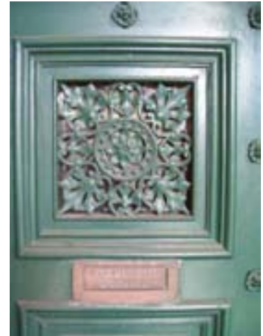
Figure 29: Cast iron vent in the entry door to the Legislative Council Chamber
