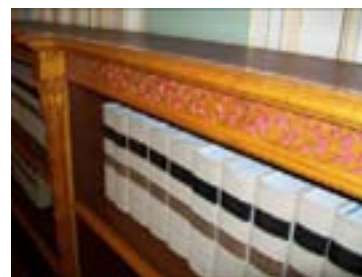
Figure 211: Bookcase in the Legislative Council Chamber with fretwork and cedar shelves faced with yellowwood
