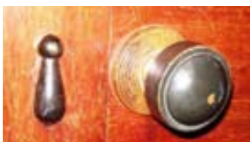
Figure 180: Handle possibly used as an early replacement for the ebony handles and roses. The tear drop shape escutcheon probably dates from 1880–1915 35 .
