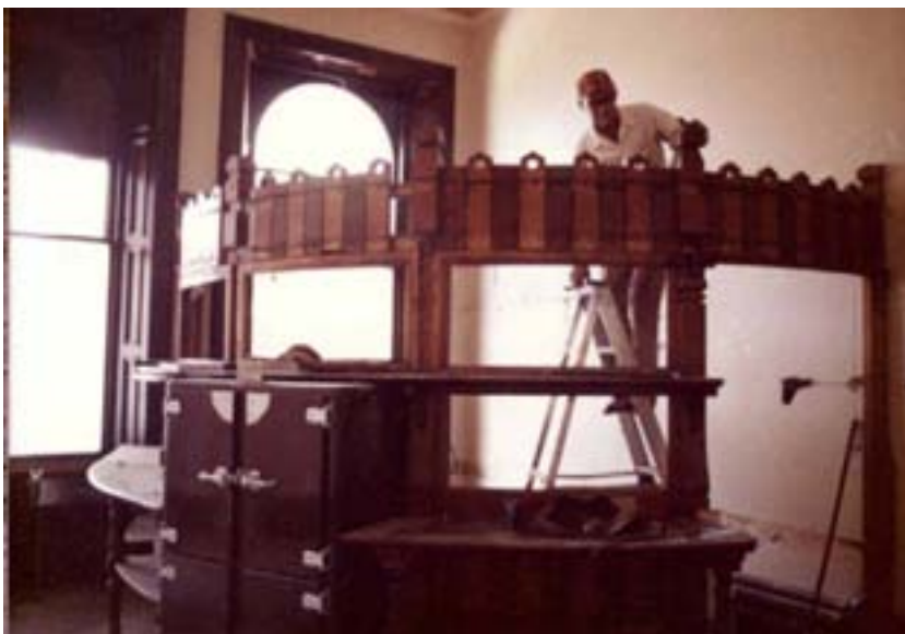
Figure 93: The curved bar being dismantled for relocation
