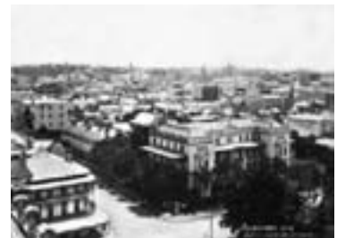
Figure 10: View from Parliament House, 1898, showing the Queensland Club and part of the former Bellevue Hotel
