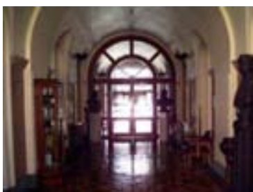
Figure 166: The carriage way is now enclosed with glazed screens and a tiled floor has been added
