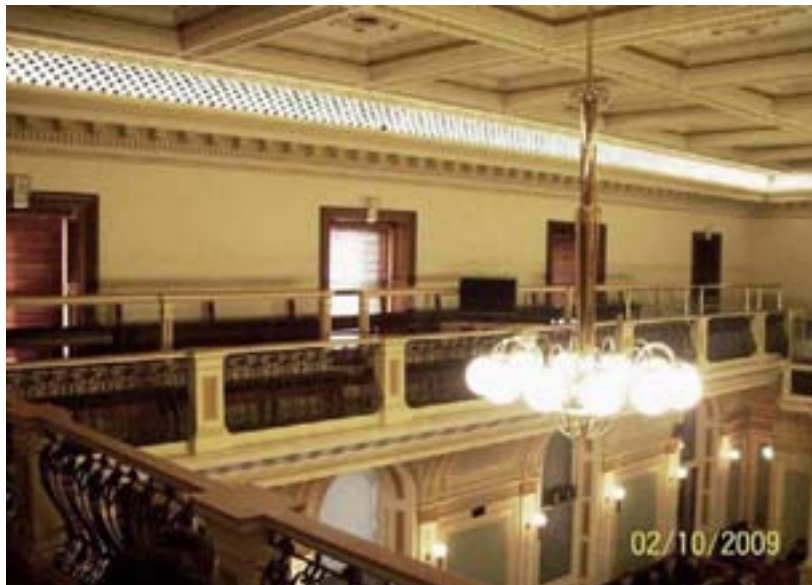
Figure 125: Legislative Assembly Chamber galleries with raised platforms and new railing behind the original balustrade. The light fittings are new.
