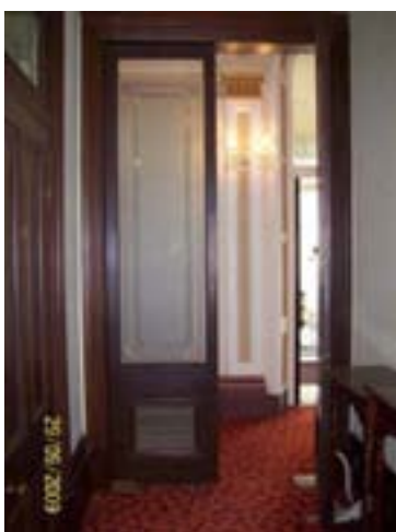
Figure 130: Anteroom doors, which have new etched glass and louvred panels
