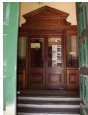
Figure 177: The main Alice Street entrance. The joinery detail echoes aedicules in the main entrance lobby from George Street
