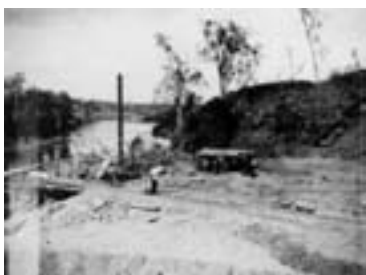
Figure 14: Quarry works at Darra on the Brisbane River, 1915, an example of a riverside quarry
