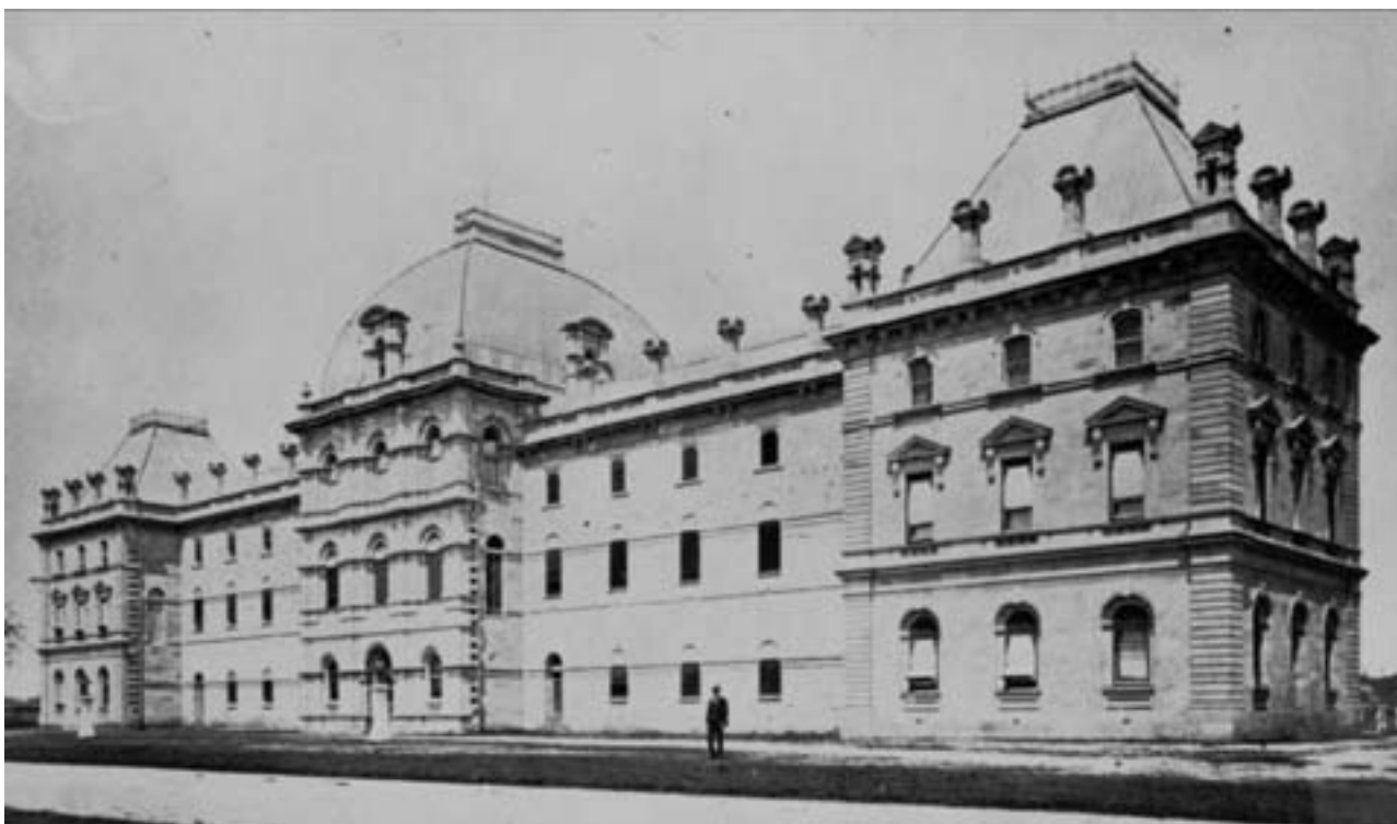
Figure 17: Parliament House, ca.1869. The photograph shows that the arcades were yet to be added however the keyed stonework and recesses for framing the roofs were already in place, along with French doors leading from the President's office and the library on the first floor. The cast iron cresting on the roof has been added and the stone pinnacles, some of which were chimneys, have been installed on the parapet. Blinds have also been added: those on the side towers are probably patent 'Florentine' blinds with timber valances, while the blinds elsewhere are dark coloured vertical sliding shutters. The roof was originally to be of slate, of similar colour to the zinc that was finally used.
