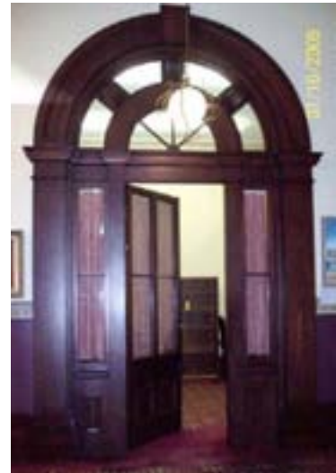
Figure 176: Doorway from the eastern entrance lobby into room A24, originally a waiting room. There is a similar doorway at the other end of the wing. The waiting rooms provided access to the reporter's stairs leading to the galleries.
