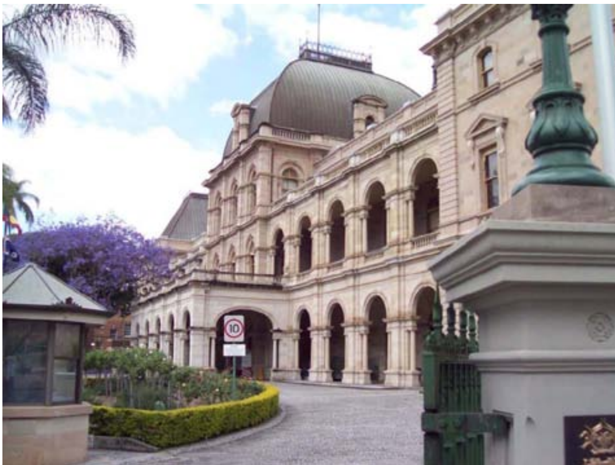
Figure 98: Parliament House from the north, showing Charles Tiffin's George Street wing of 1865–68 with arcades added in 1878–79. The porte-cochere, guard house and granite set paving were added in the 1980s.
