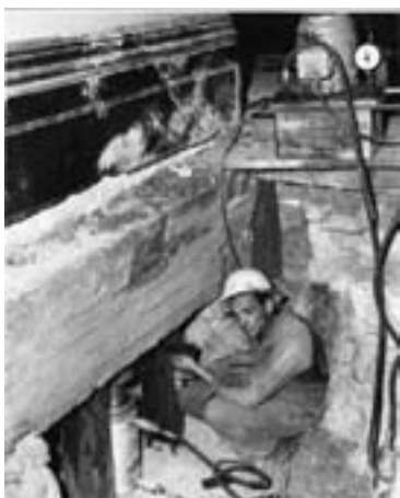
Figure 66: Underpinning Parliament House in 1969
