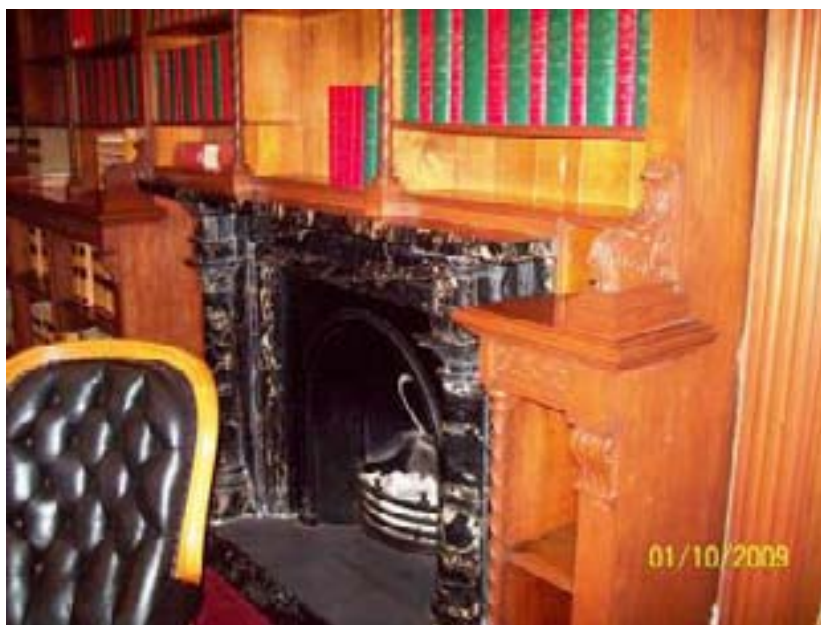
Figure 138: Chimneypiece of opulent Potoro marble in the first floor Library
