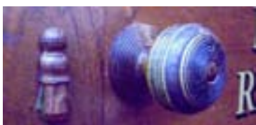
Figure 179: Reeded timber handles are evident in two forms: domed, like this one, and flat
