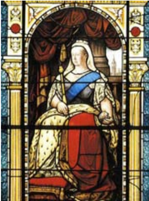
Figure 185: Detail of the Queen Victoria window, new lead comes have been used to repair breaks in the glass
