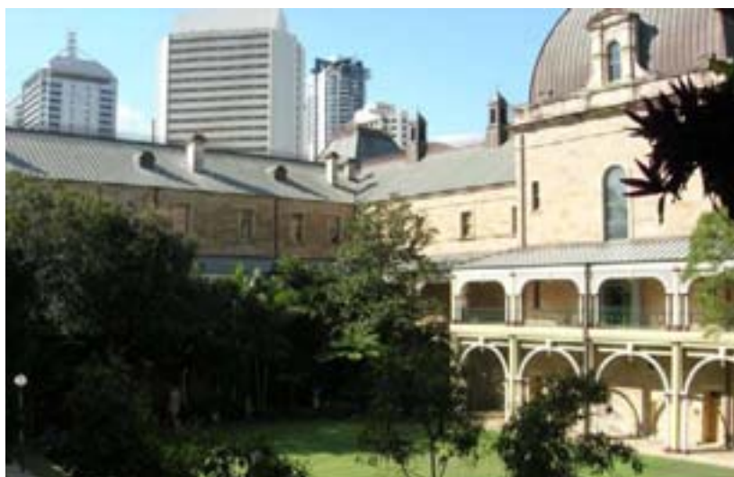
Figure 118: View from the Annexe with the Speaker's Green in the foreground. There are no parapets on the back walls consistent with the plainer character of the courtyard elevations.
