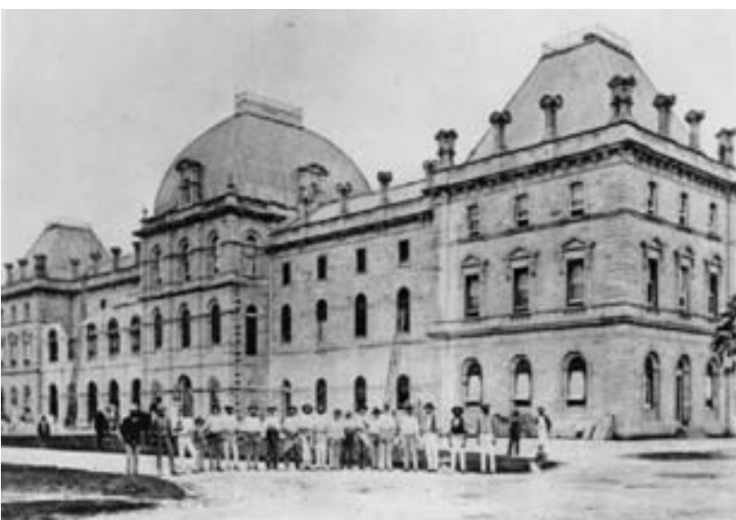
Figure 32: John Petrie's workmen during construction of the arcades, 1879
