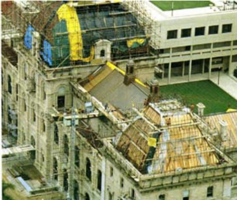
Figure 88: Installing the new roof sheeting
