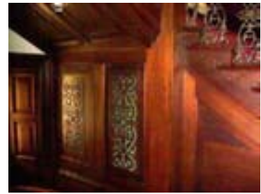
Figure 171: The cedar casing on the grand staircase at ground floor level incorporates fretwork panels
