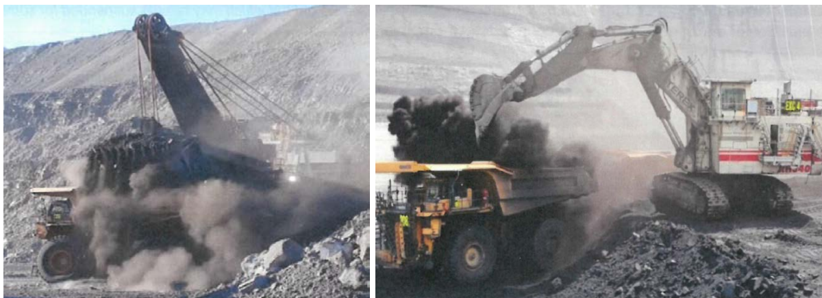
Image 12 Dust generated by machinery in an open-cut environment
