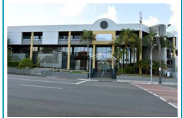
Construction starts on the new Woolloongabba Community Health Centre which will be home to public Oral Health and Addiction and Mental Health Services
