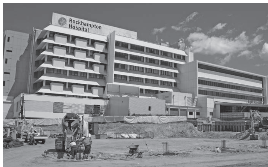
photo: construction zone, Rockhampton Hospital
