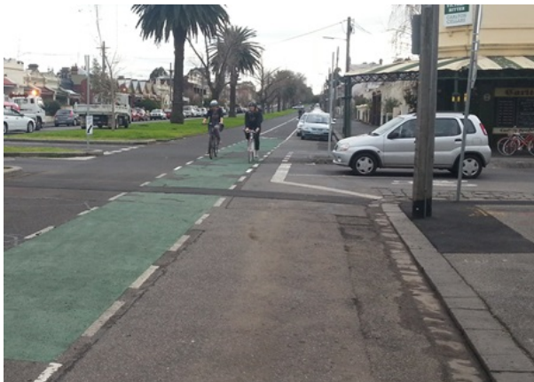
Figure 27 Example of advanced Stop/Give Way line marking and parking set back distance to provide clearer line of sight at minor intersection. 414
