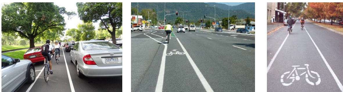
Figure 25: Examples of on-road separated bicycle lanes which meet design standards 380
