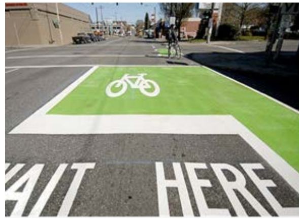
Figure 28 Example of advanced stop line (bicycle storage box) at signalised intersection. 415
