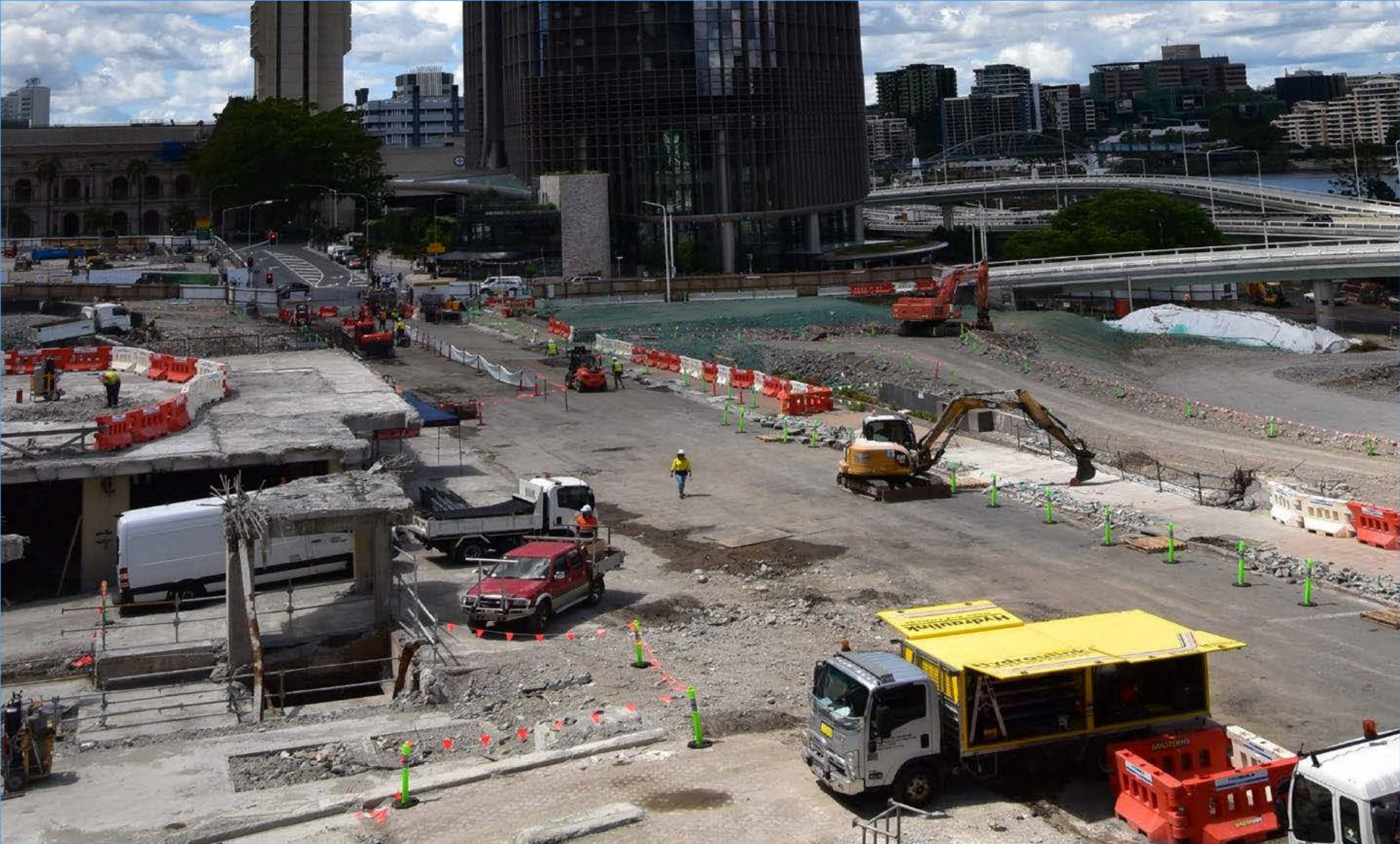
William Street site prior to 2018 excavation
