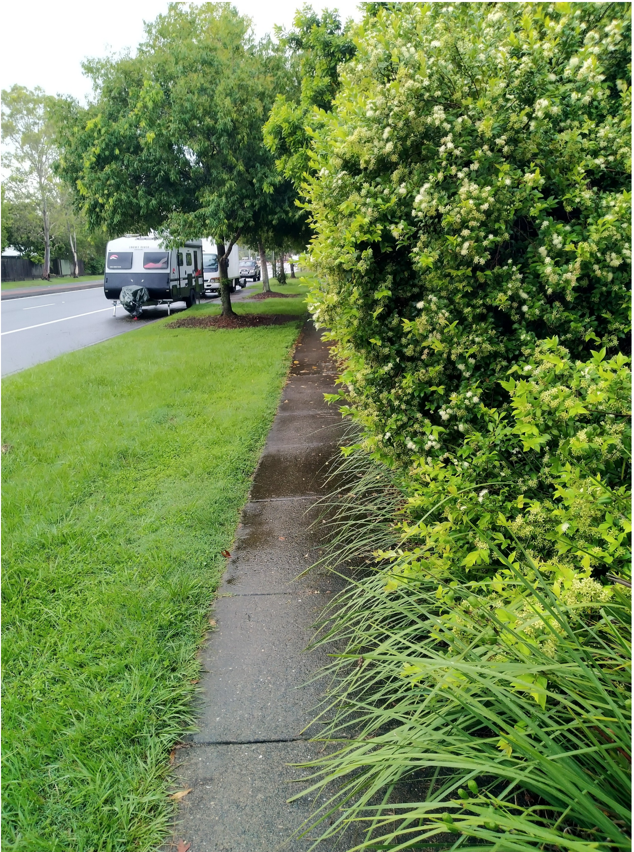
3. A little further along Albany Creek Road in Aspley – a medium-density residential area with several retirement and aged-care facilities – pedestrians, cyclists, and PMD users are expected to all share this minimum-width footpath, made even narrower by overhanging ornamental vegetation,
