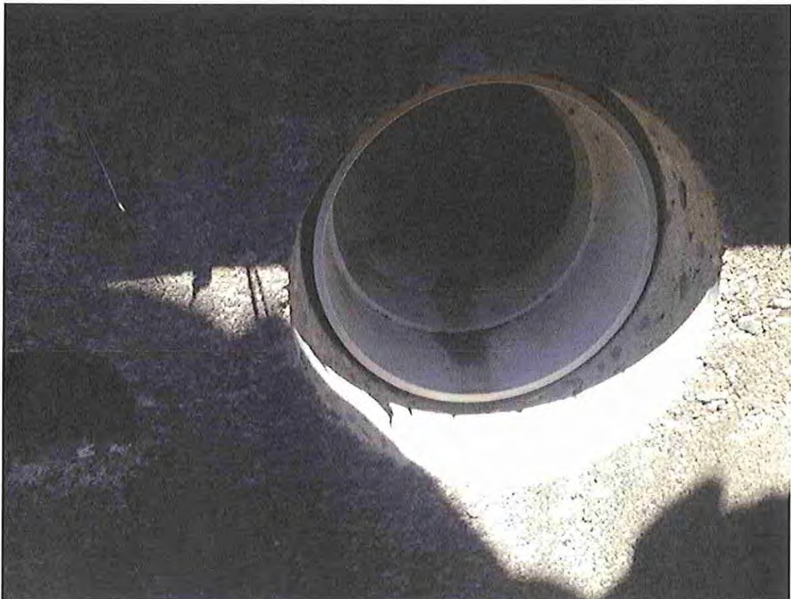
Inside stormwater drain, pipe which is connected to sewer
