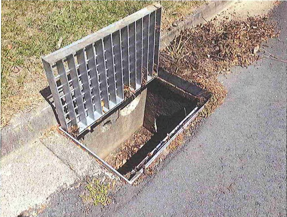
Stormwater drain on Orchid St, Redcliffe (shows pipe coming from sewer)
