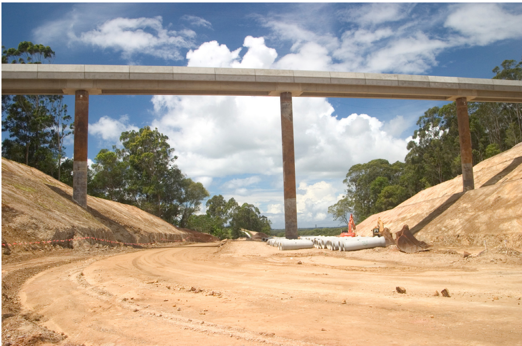
Figure 3: Tugun Hill Bridge looking south
