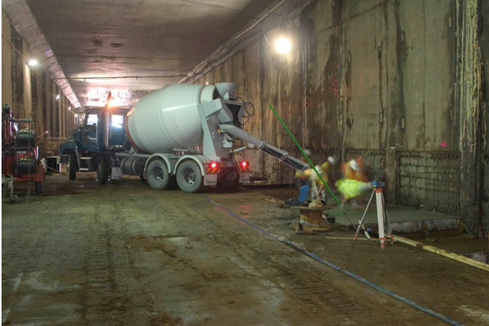
Figure 3: Completing blinding layer for concrete floor in the tunnel
