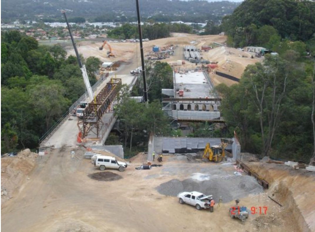
Figure 2: Construction of Hidden Valley bridges
