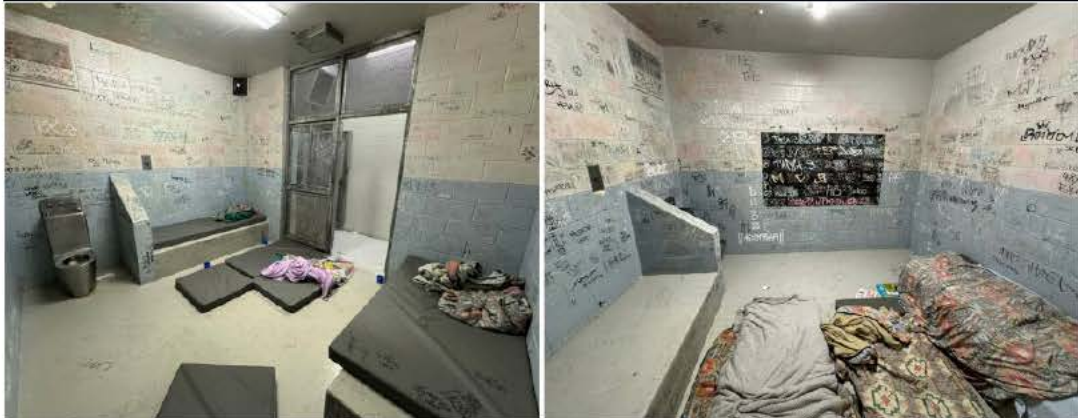
Figures 1 and 2: Accommodation cells in the Boys' unit at the Cairns watch house (Sept 2024) 31
