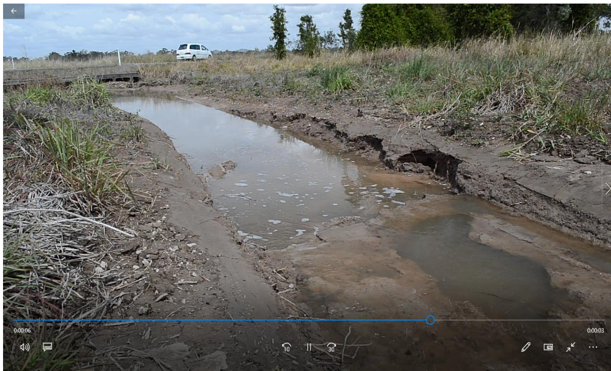
Fig. 11 (d) Eroded cane drain flowing to the clogged underpass under the Bruce Highway (sept 5 th 2018). Dissolved Inorganic Nitrogen (DIN) levels 9 times the limit in cane drain runoff.
