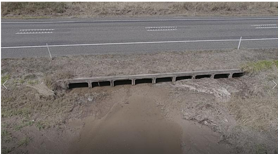
Fig. 11(e) Cane drain sediment-laden runoff under the Bruce Highway and through the former Lily Creek drainage line to Clairview Estuary (Sept. 5 th 2018.
