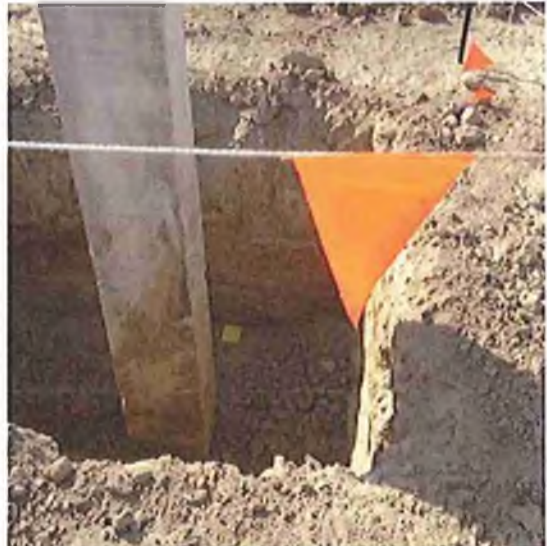
Failure to install edge protection and shoring and battering on excavation creating fall from heights and cave-in hazards
