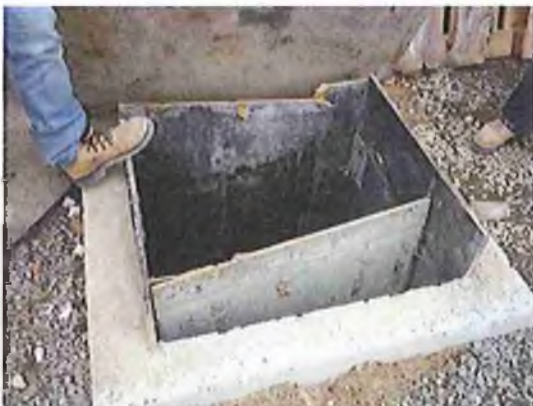
Failure to install edge protection on penetration creating fall from heights hazard
