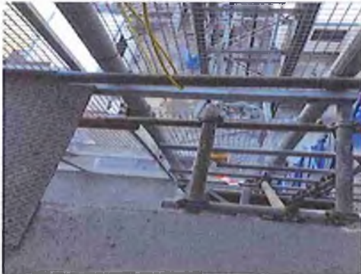
Failure to install edge protection creating fall from heights hazard
