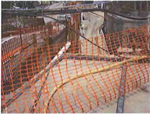
Failure to install edge protection and install complete scaffolding creating fall from heights hazard
