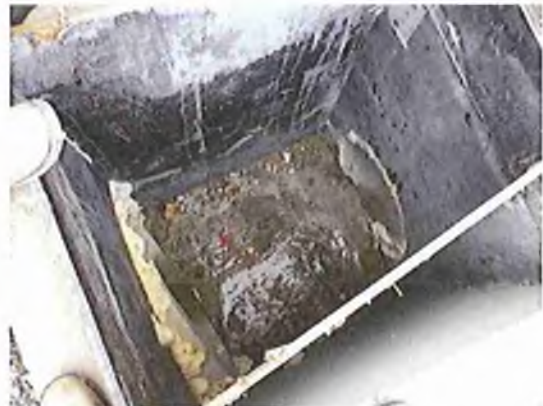
Failure to install edge protection on penetration creating fall from heights hazard
