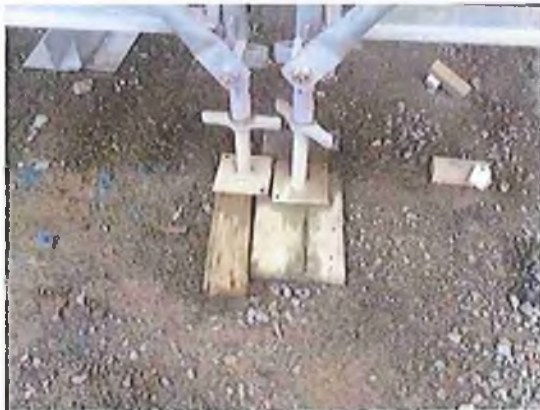
Non-compliant sole-boards creating scaffold collapse hazard
