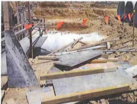
Failure to install complete scaffolding, edge protection and barricading creating fall from heights hazard
