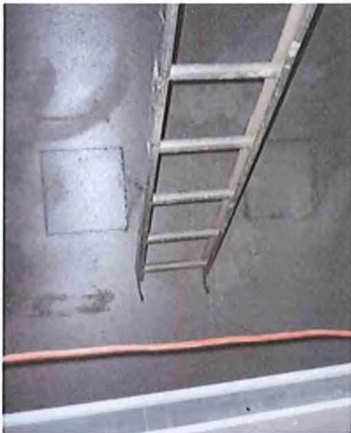
Failure to install edge protection on penetration creating fall from heights hazard
