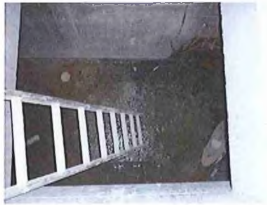
Failure to secure ladder footings creating fall from heights hazard (note markings in first photo showing where ladder has slipped while being accessed by worker)
