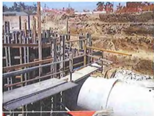
Failure to install complete scaffolding, edge protection and barricading creating fall from heights hazard
