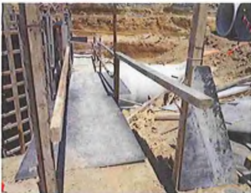
Failure to install complete scaffolding, edge protection and barricading creating fall from heights hazard
