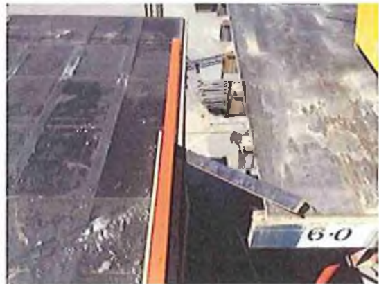
Failure to install edge protection and barricading around openings in formwork on live deck creating (note concrete finisher used adjacent to unprotected edge)
