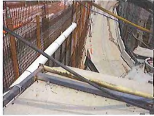
Failure to install edge protection and install complete scaffolding creating fall from heights hazard
