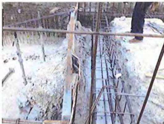
Failure to install edge protection creating fall from heights hazard
