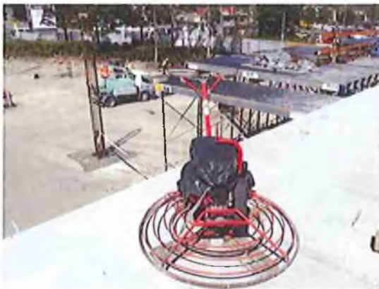
Failure to install edge protection and barricading around openings in formwork on live deck creating (note concrete finisher used adjacent to unprotected edge)
