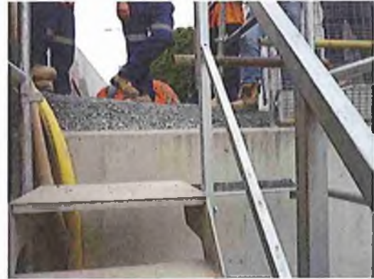
Failure to install edge protection and install complete scaffolding creating fall from heights hazard
