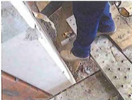
Non-compliant sole-boards creating scaffold collapse hazard
