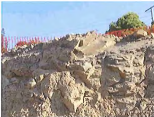
Failure to install edge protection and shoring and battering on excavation creating fall from heights and cave-in hazards
