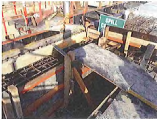
Gap in scaffolding greater than permitted by regulations creating fall from heights hazards
