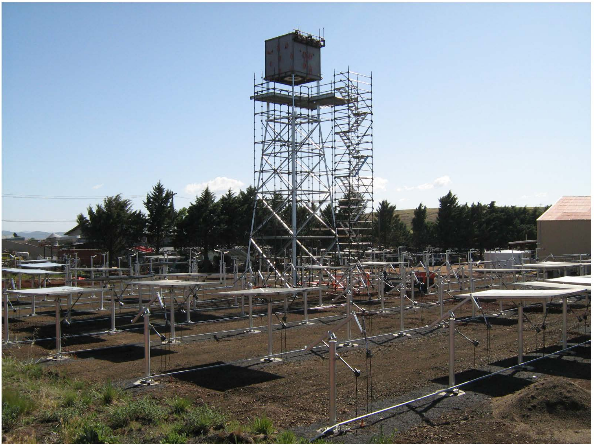
First module being prepared for demonstration in Cooma NSW
