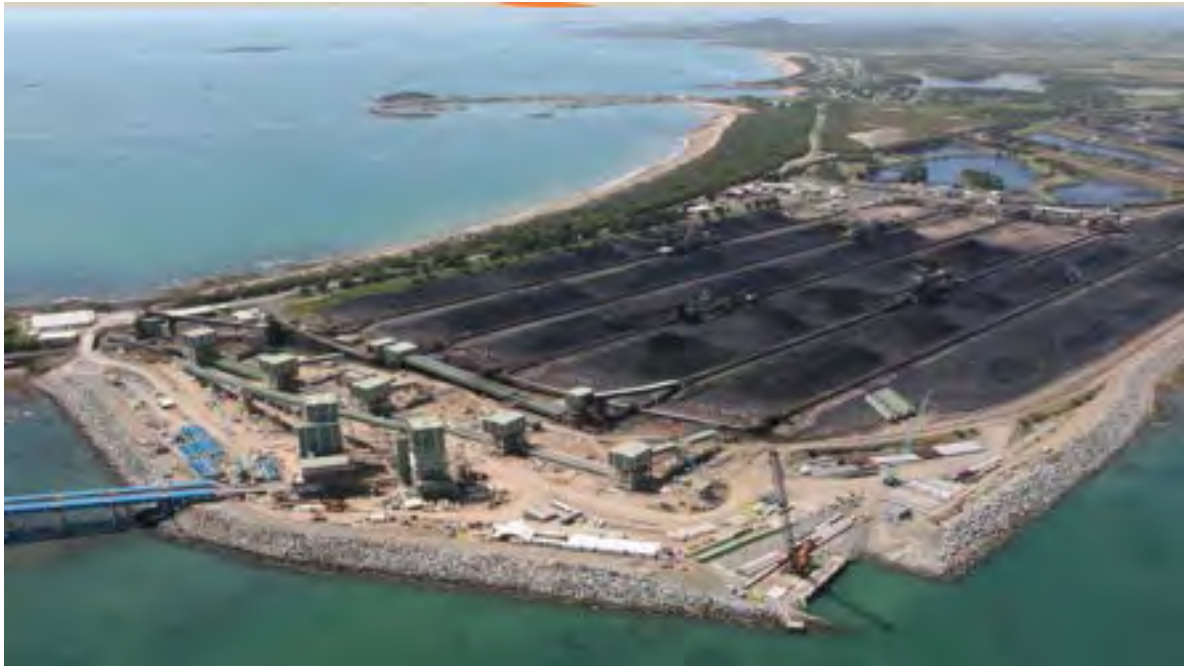
Figure 2. Hay Point Coal Terminal
