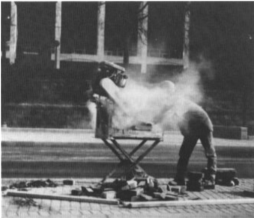
Figure 7: Cutting bricks
