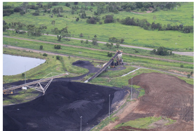
The Sonoma Coal Mine CHPP beside the road.
