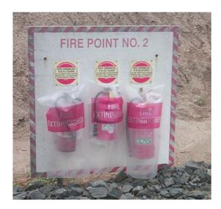
Figure 9: Fire fighting equipment clearly accessible inside the magazine perimeter
