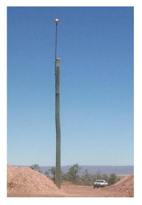
Figure 7: Vertical conductor used to protect relocatable steel magazines
