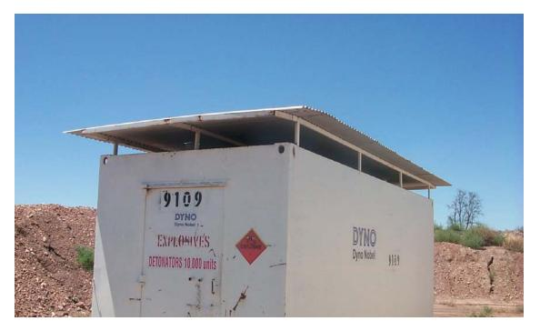
Figure 6: Shade roof on a steel relocatable magazine
