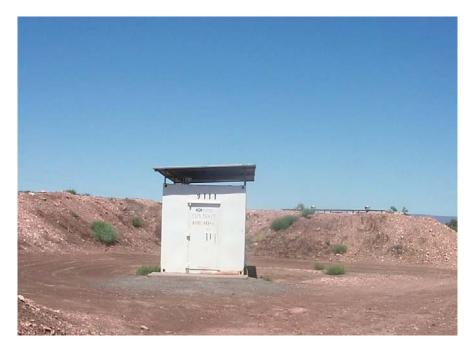
Figure 2: Relocatable magazine protected by earth mounds
