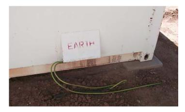
Figure 8: Earthing terminations on a steel relocatable magazine
