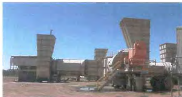
Figure 4. Coal mine main fan and duct system on shaft.
