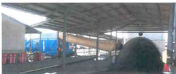
Figure 16 - Suitable location for real-time air velocity measurements to carry out performance evaluation of Bulk Air Cooler (BAC)
