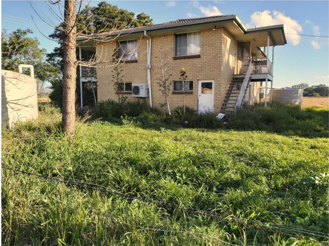
Current condition of rental house
