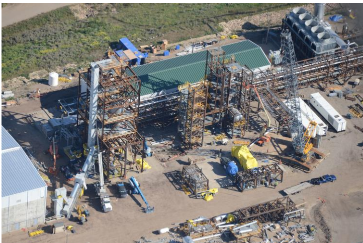
Figure 4: Enerkem MSW to Ethanol Plant in Alberta Canada
