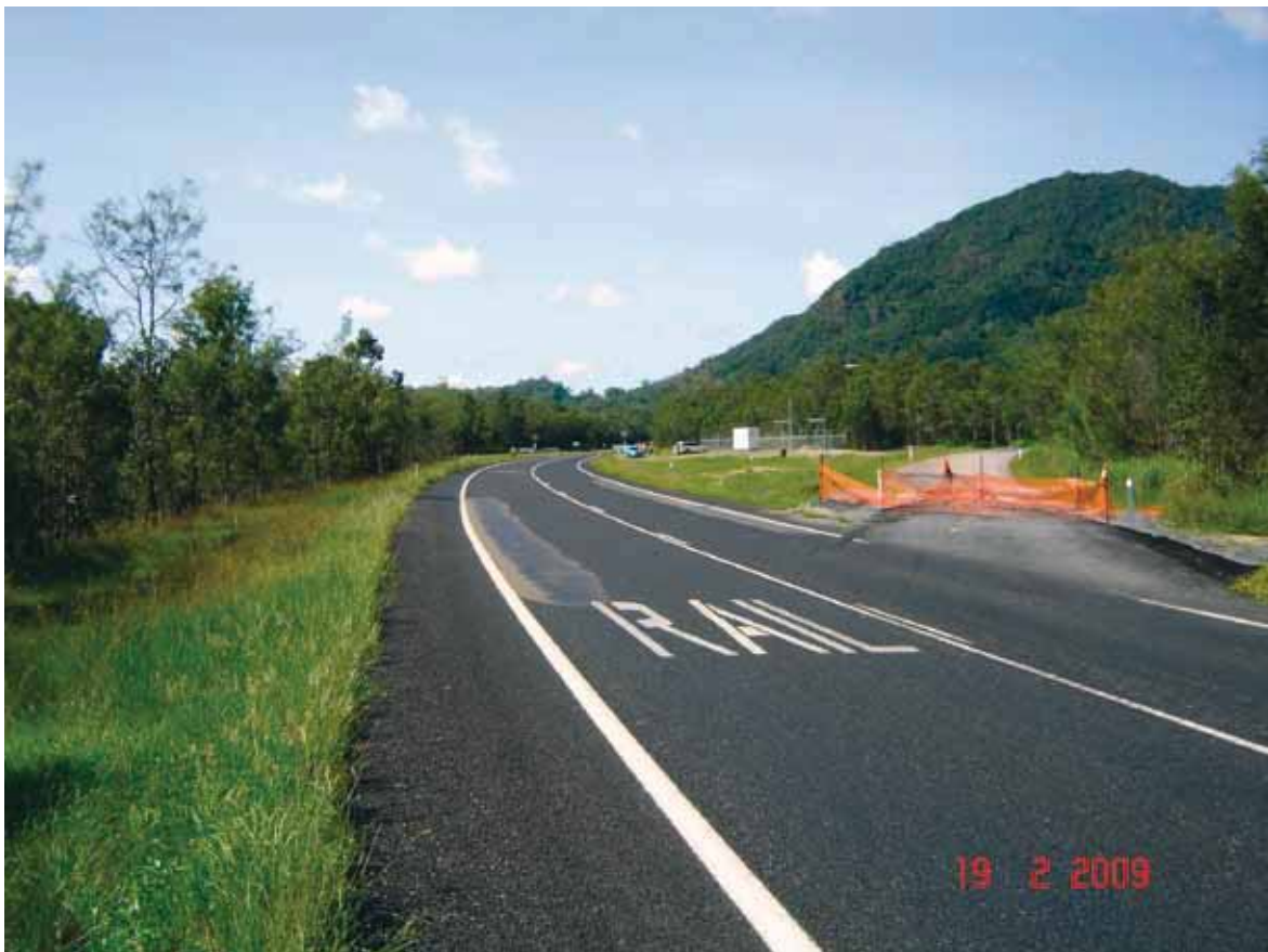
Figure 3: Approach to the level crossing from the north
