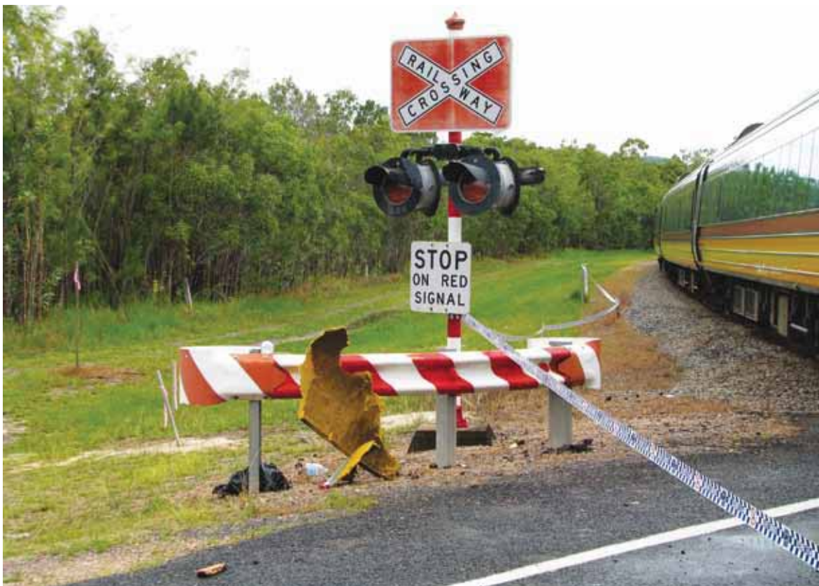
Figure 28: RX 5 level crossing signal assembly Rungoo crossing (northern)
