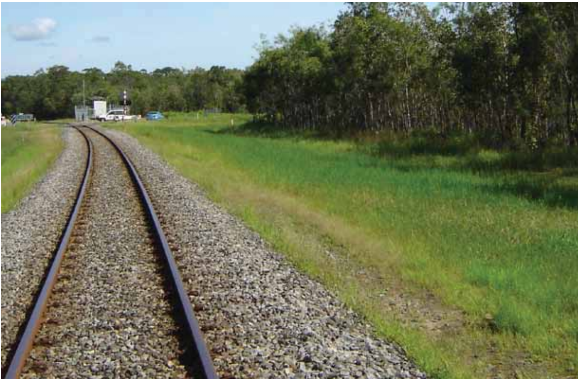
Figure 25: View from track, about 100 m from crossing
