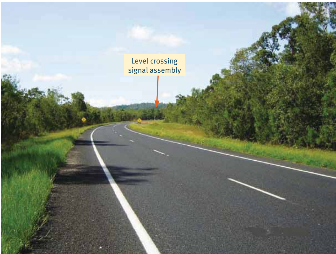
Figure 30: First sighting of level crossing signal assembly (Southbound)
