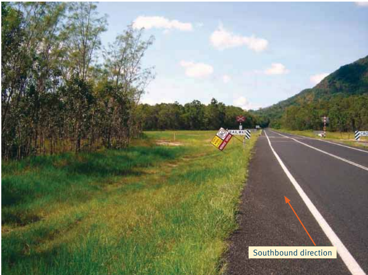
Figure 34: Restricted view of rail line, approach to Rungoo level crossing
